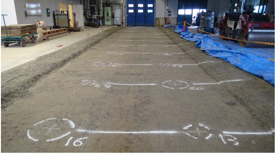
Figure 2.1.3: Compacted surface with marked PLT measurement locations before further testing.
